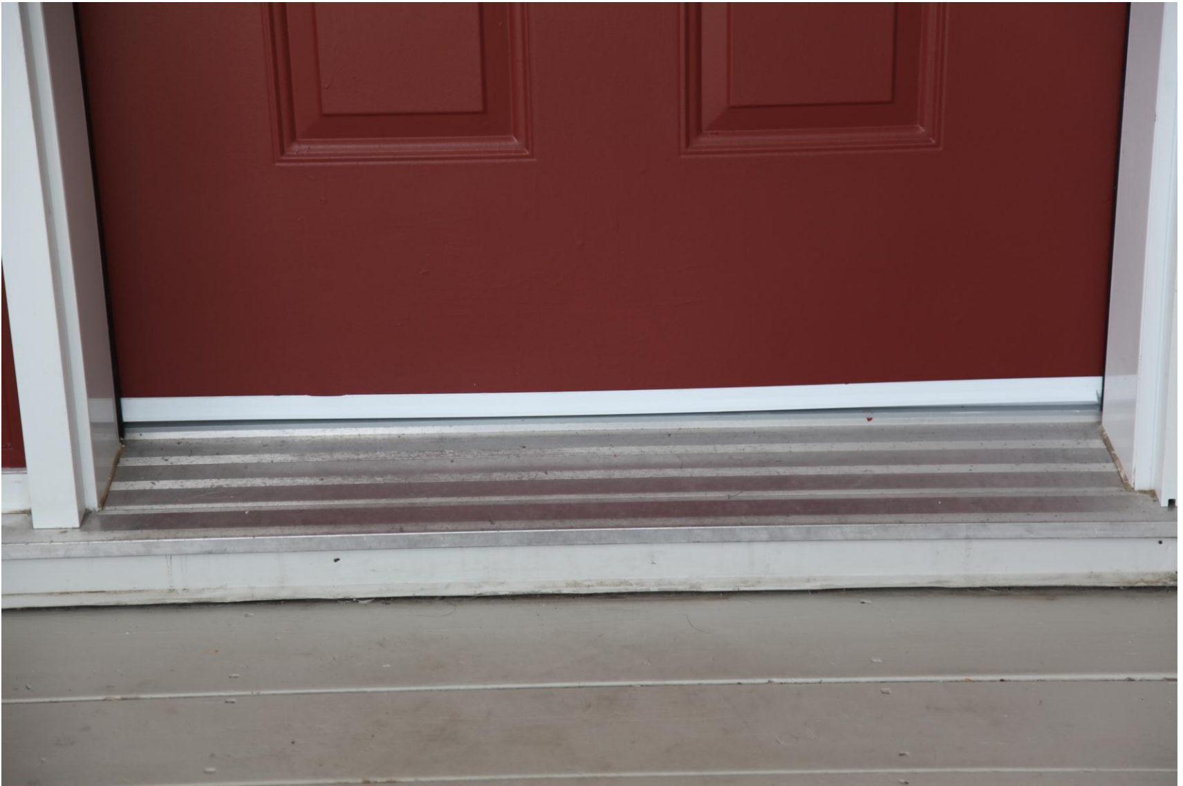
New door Threshold keeps drafts and snow outside not blowing inside.
