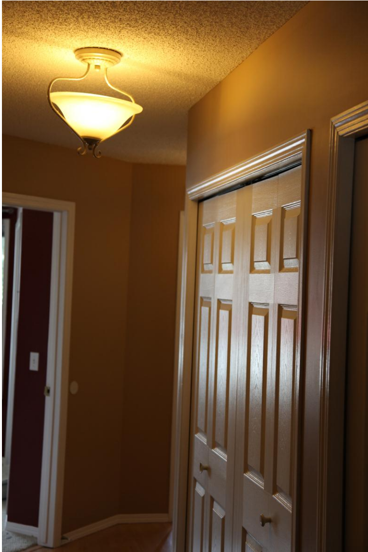
Light fixtures fastened and hallway doors gleaming with a fresh coat of paint.
