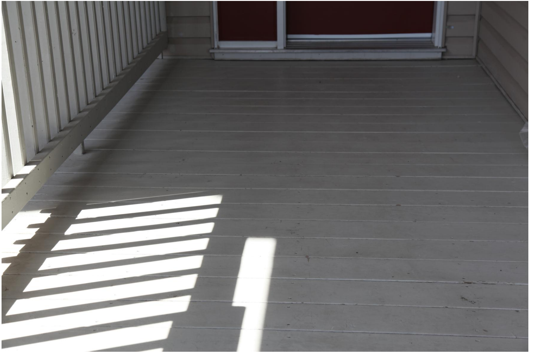
Front Veranda scrubbed clean.
