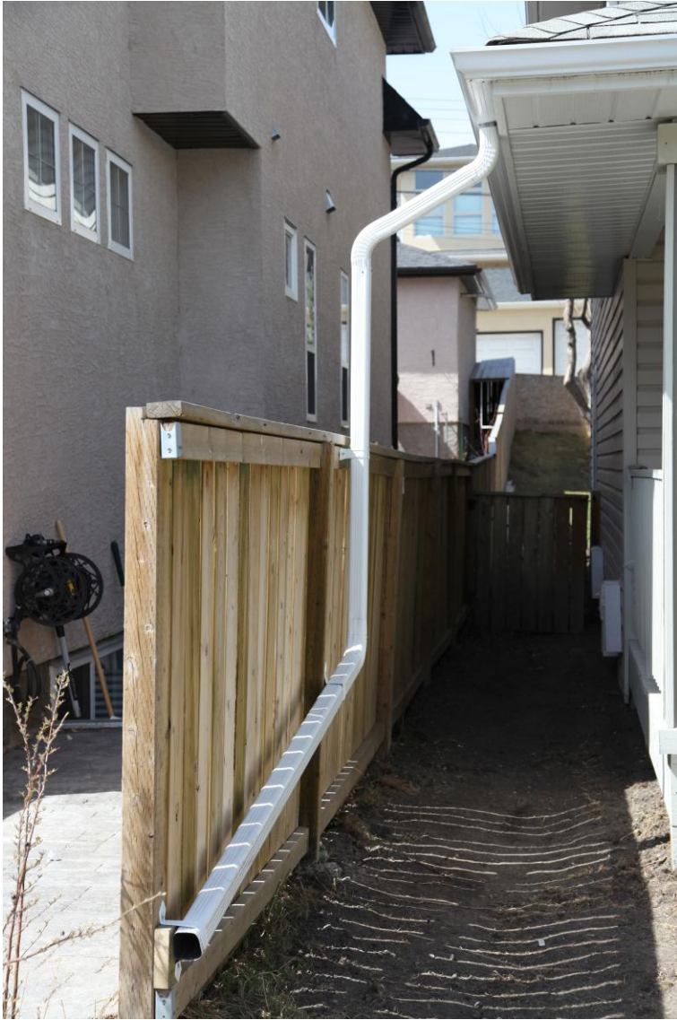
New installation and re-positioned drain spout means no more ice hazard at front step.
