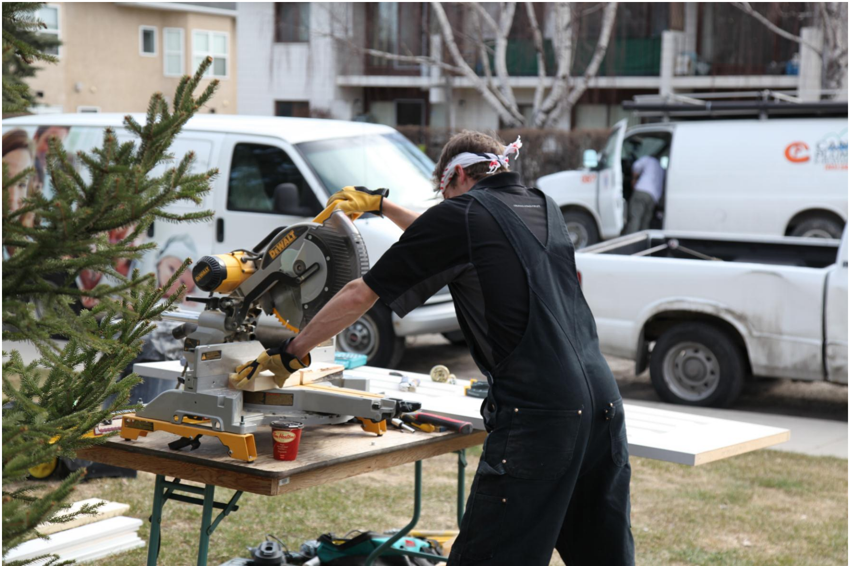
Johnnie getting blocking prepped to lift those Sidewalks in place!
