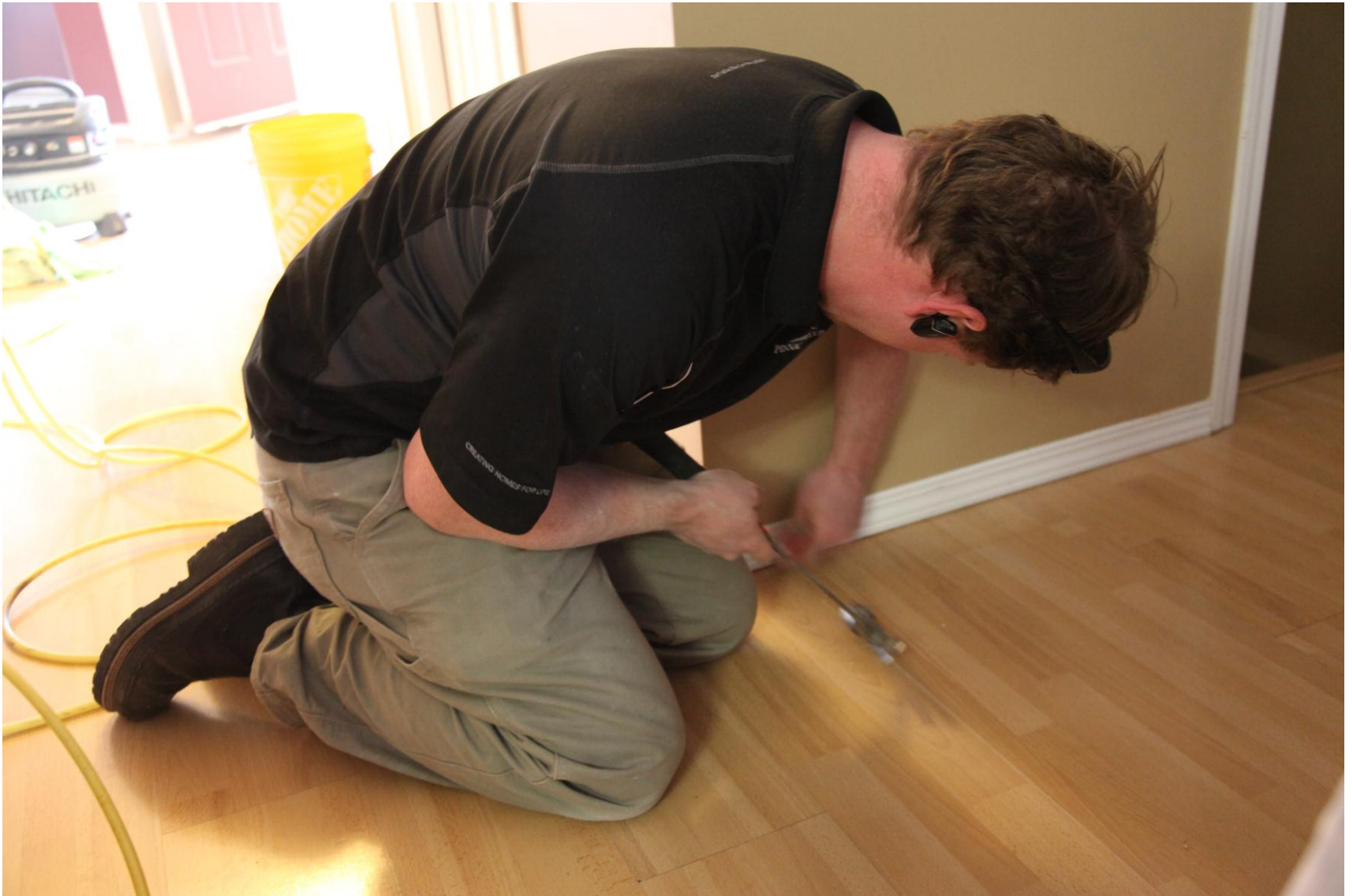
Brennan repairing millwork pre-paint!
